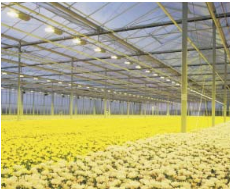
The most used lamps for supplementary growth lighting are high pressure sodium lamps.
