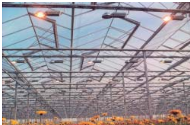
Plant photosynthesis is determined by the number of photons between 400 and 700nm, in natural light or emitted from artificial lights, which are absorbed by the leaves.
